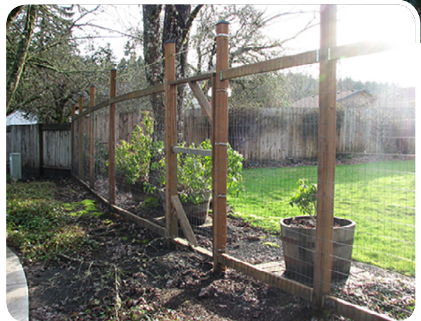
Top: An improvised and failed deer fence Bottom: An effective and attractive urban deer fence along a common area
