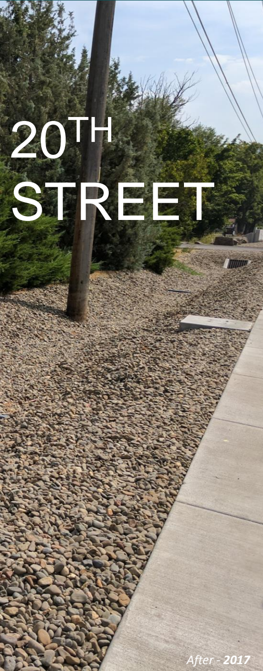
Figure 1. As stormwater flows through the swale, the flow spreaders, (sometimes called check dams) will act as ponding agents, slowing the release of water. The flow spreaders have a 1" maximum exposure over the bottom of the swale and are secured with stakes.
