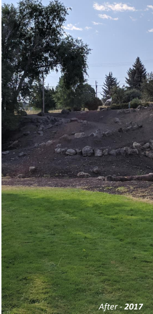
Figure 1. This vegetated filter strip receives sheet flow from a street and slowly directs runoff into a perforated pipe which then connects to the water quality conveyance swale.
