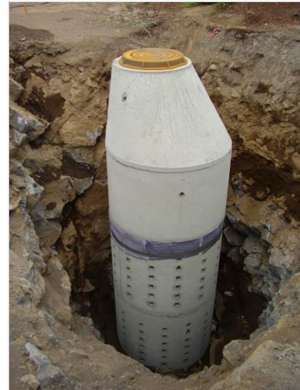
A drywell under construction.
