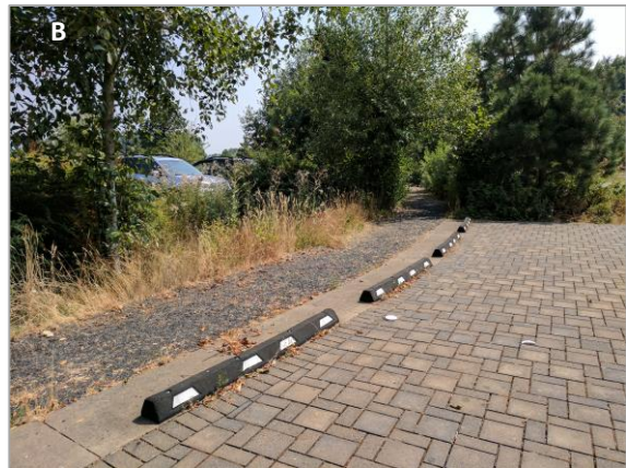
A. Porous Concrete and Share a Driveway BMP. B. Permeable Pavers and Permeable Gravel paired with an Infiltration Rain Garden.
