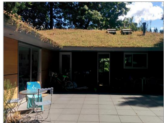
Residence with a vegetated roof. Consult with a structural engineer to be sure that installing a vegetated roof is feasible.
