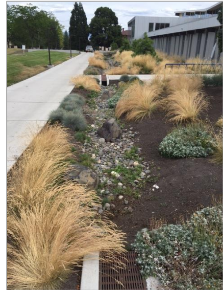
Water Quality Conveyance Swale
