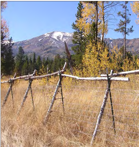
Figure 56. Poletop panel fence type. (Photo: N. Christoffersen)
