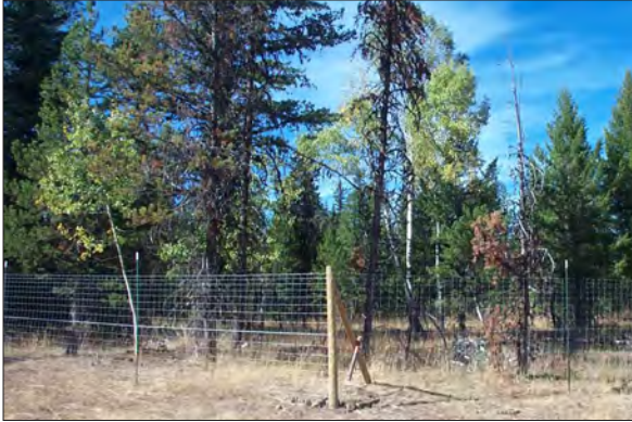
Figure 54. Woven wire fence type. (Photo: N. Christoffersen)
