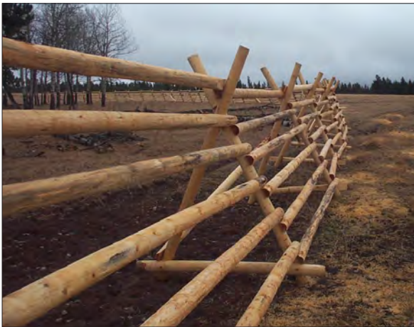
Figure 55. Buck and pole fence type. (Photo: N. Christoffersen)
