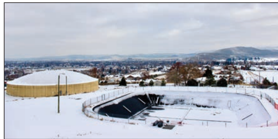
Photo: Emily Jane Davis, © Oregon State University Figure 9-10. Water storage infrastructure.
