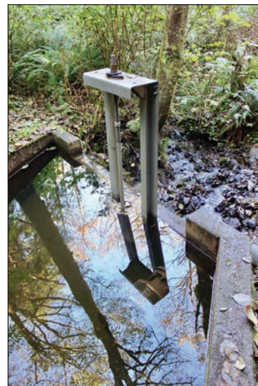
Photo: Emily Jane Davis, © Oregon State University Figure 9-14. Current intake on Coleman Creek for Cape Meares treatment plant.
