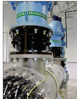
Photo: Emily Jane Davis, © Oregon State University Figure 9-11. A component of the UV treatment system.
