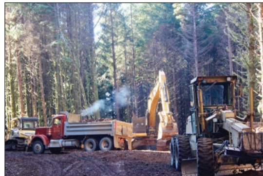
Photo: Emily Jane Davis, © Oregon State University Figure 9-12. Improvement of forest road on Stimson timberland for future harvest operations
